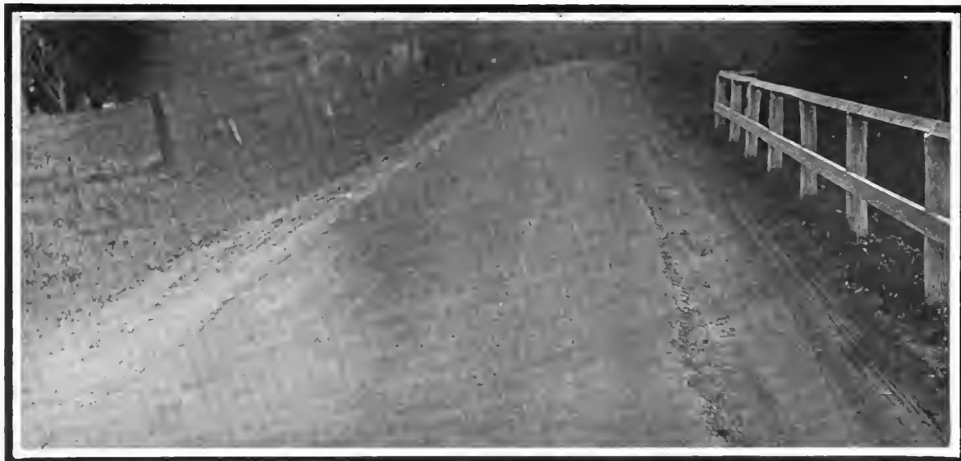
Two-thirds of this road is crowned so stiffly that horses are forced to the right. It is three years old
